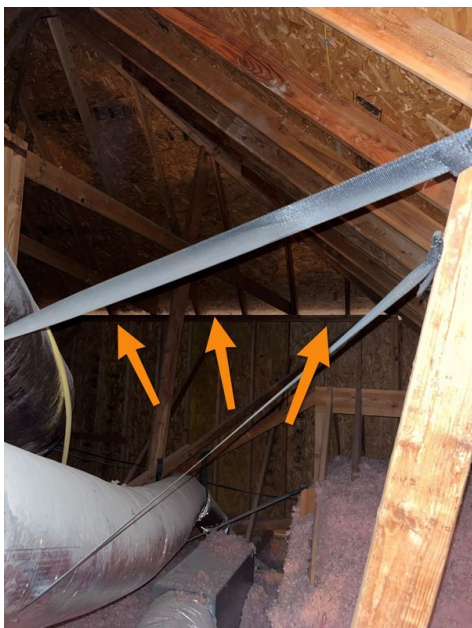
Soffit venting
