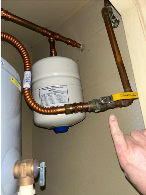
Shut-Off & Expansion Tank
