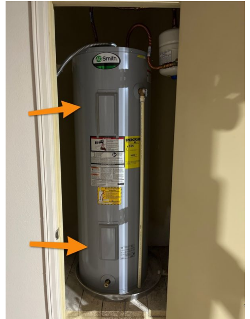
No Seismic Bracing
