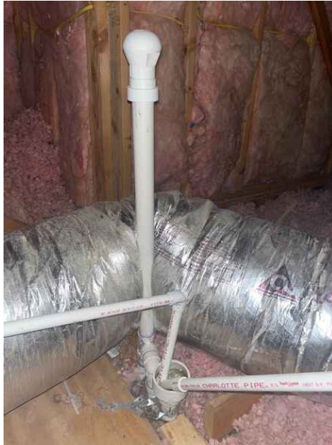
Into open, trapped drain
