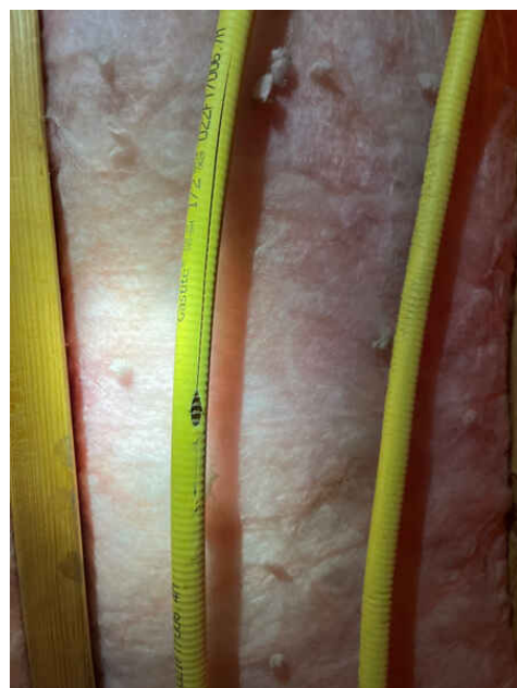
Damaged sheath
