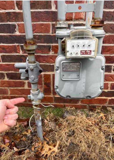
Main Gas Shut-Off Location
