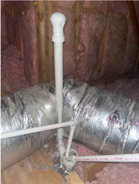
Into open, trapped drain
