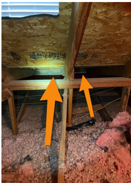
Soffit venting
